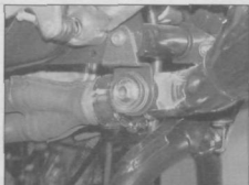
13.6a Exhaust system is retained by a bolt to the frame ...
