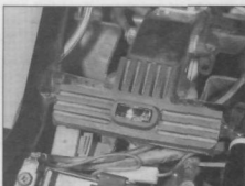
2.8 Inspect the rubber mount at the rear of the tank
