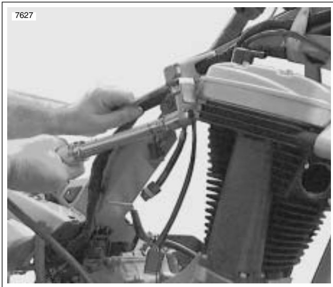
Figure 3-38. Install Top Rear Tie Bar
