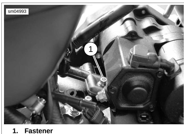
Figure 3-31. Return Oil Manifold
