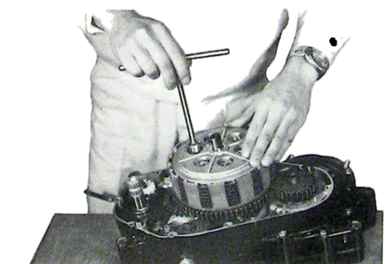
Fig. 5-1-7 Loosening clutch spring bolt
