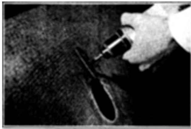
Figure 2-55. Rough Sanding Inside Surface
