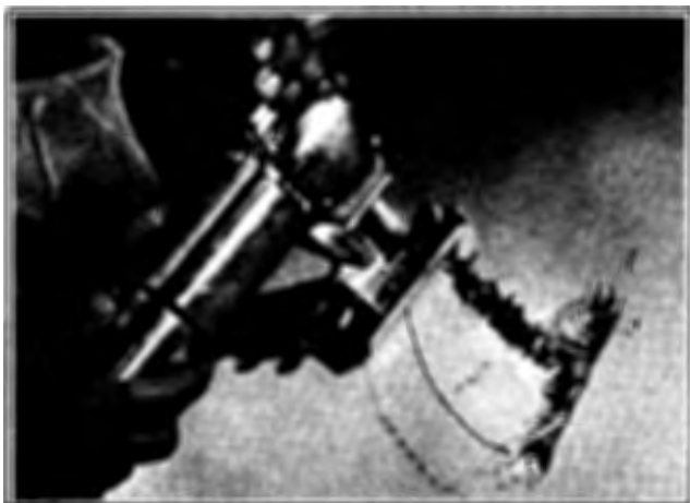
Figure 2-54. Sawing Out Damaged Area
