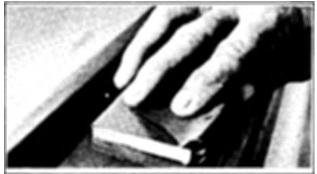
Figure 2-53. Sanding Patch
