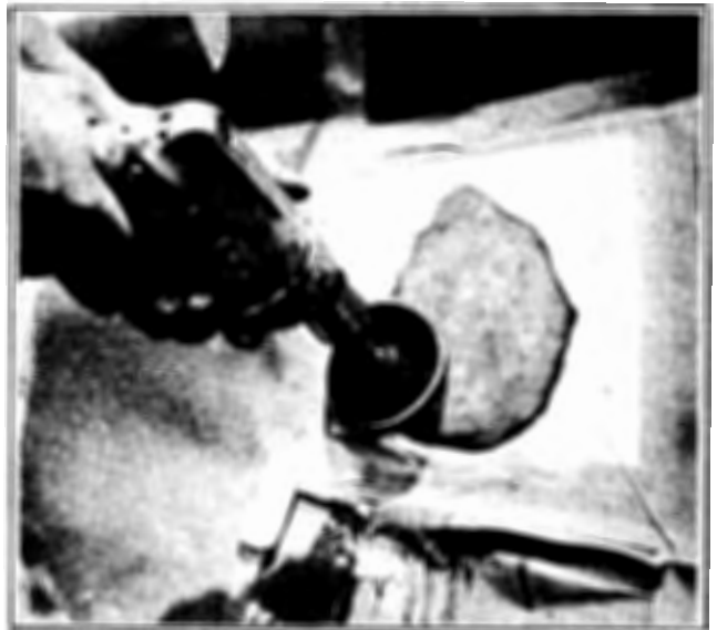
Figure 2-60. Bleeding Patch with Sander
