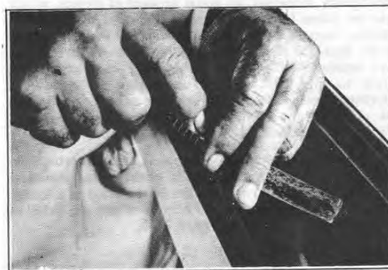
Figure 2J-4. Trimming Patch
