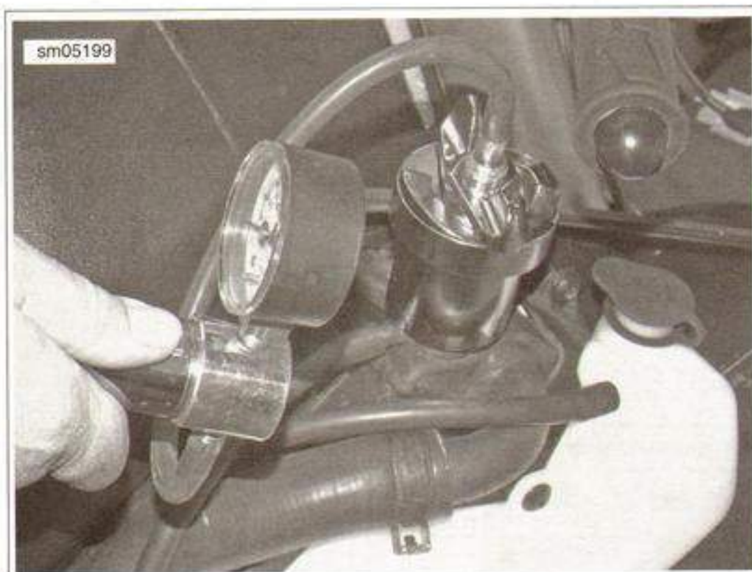
Figure 5-5. System Pressure Test
