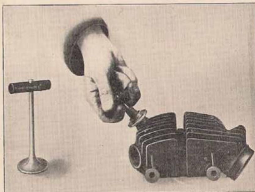
FIG. 39. THE A.J.S. VALVE GRINDING TOOL
