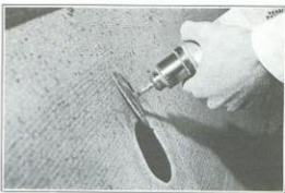
Figure 2J-8. Rough Sanding Inside Surface
