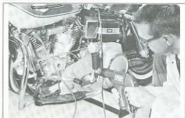
Figure 5F-3B. Checking Timing with Strobe-Lite
